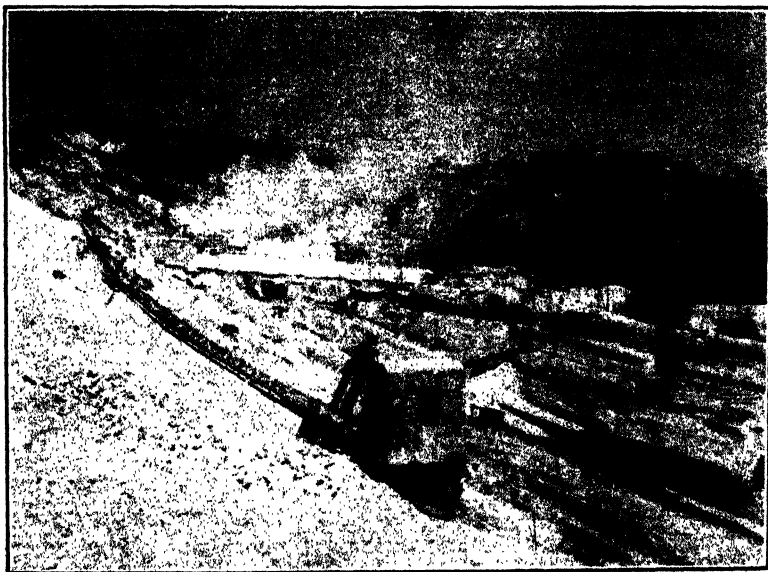
FIG. 2.—View in Diatomite quarry, Lompoc, Calif., showing machine cutting bricks from solid. ( H. Ries, photo. )
